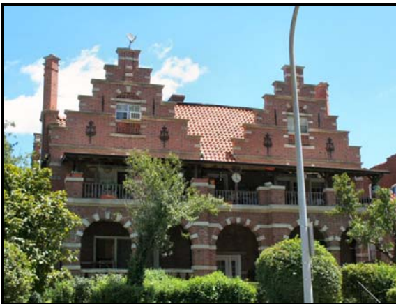
MATTIE JOHNSON APARTMENT BUILDING
