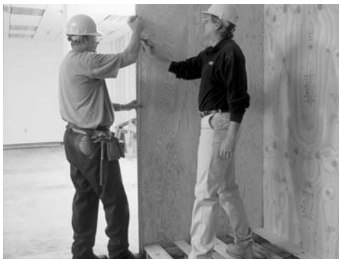
Many crews speed up the stacking by building a simple two-sided, free-standing frame. Note: Frame is not attached to pallet.
