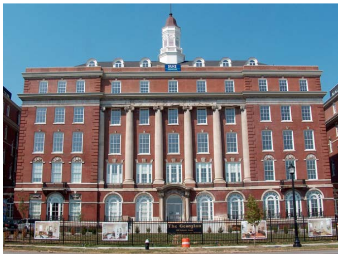
After: Restored exterior of the Georgian Condominiums.
