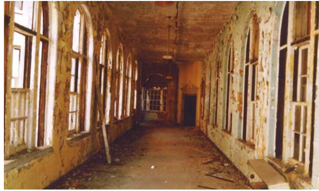
Before: Interior corridor of City Hospital administration building prior to renovations.
